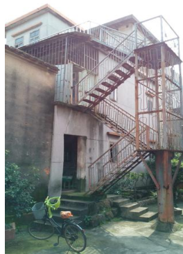
Figure 13: Additional steel ladder.
