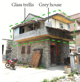
Figure 8: Balcony extending out of the roadway.
