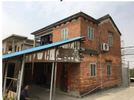
Figure 2: Red brick house.
