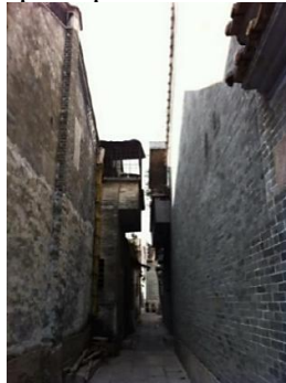
Figure 7: Balcony extending out of the roadway.
